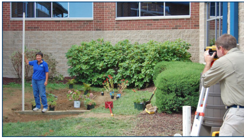
Figure 7. Anchor one end of line flat on the weir and check elevation of all upslope rain garden borders. Weir should be lowest elevation. When using a line level, the bubble should always move away from the weir.
